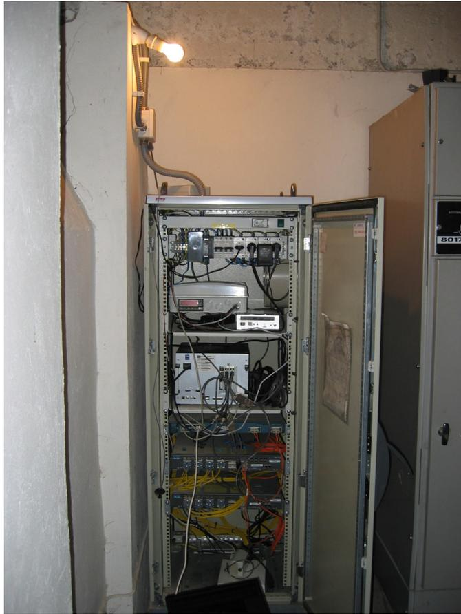
**Figure 2-5: OSGi Server in the Transformation Center's Rack**
